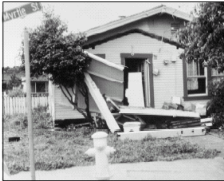
Houses that aren't bolted to their foundations shift off them.
