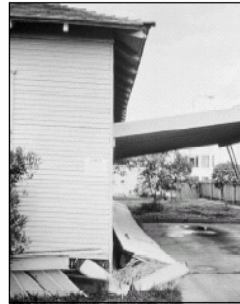
Unbraced cripple walls collapse.
