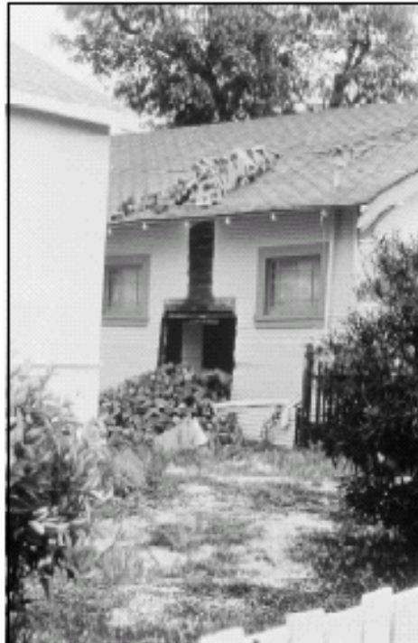
Chimney collapse is a widespread problem.
